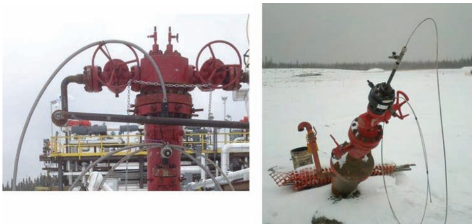
Figure 12.12 Field installation of fiber optic sensors (courtesy of Petrospec Engineering).
